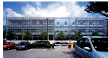
University arts & human sciences, Grenoble (France) Completion 2001 Client Université Pierre Mendès-France Program University of 1 500 students with amphitheatres, classrooms, library, administration Area 5 062 sqm Cost 3,078 M€ net
