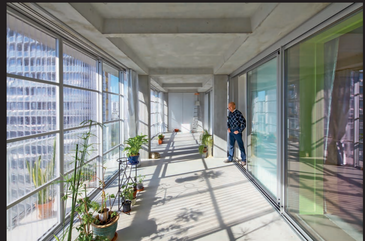
The winter gardens function as passive solar collectors and improve the energetic performance of the building envelope.
