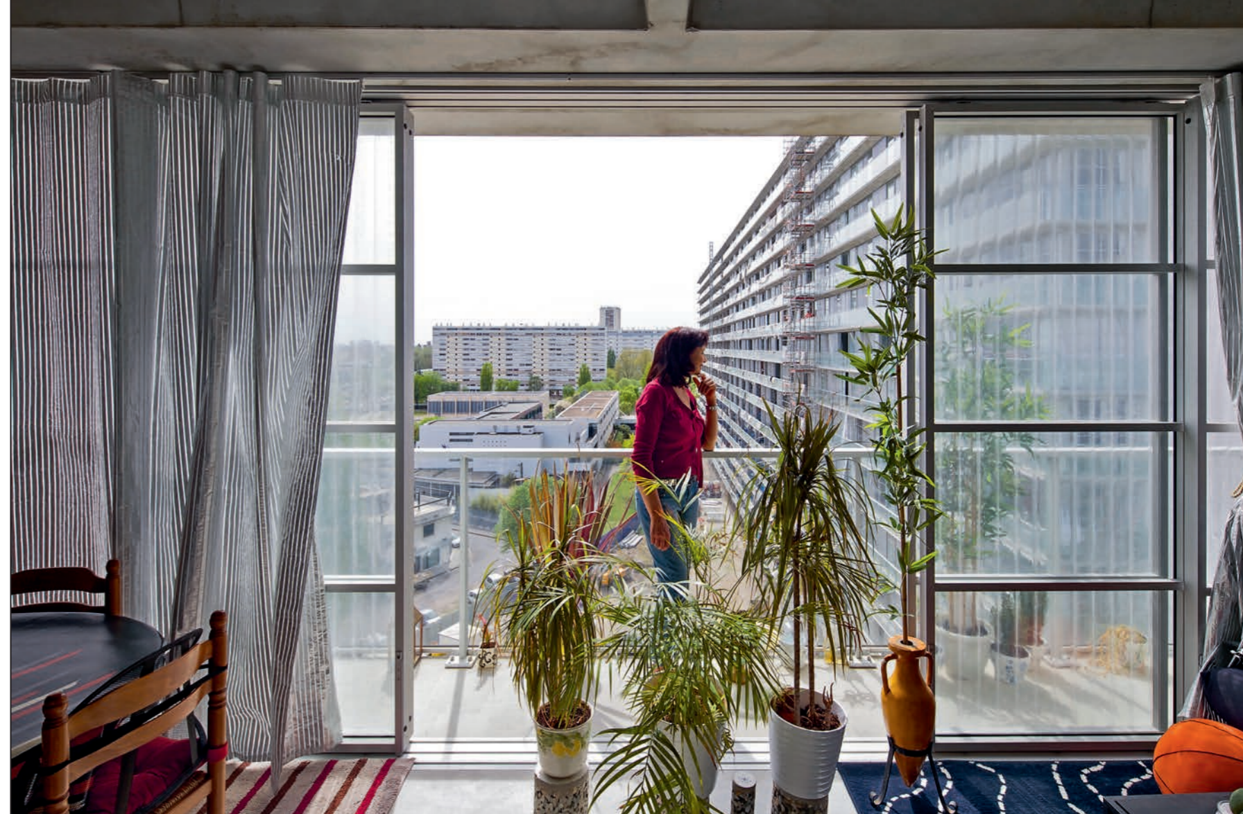
The new lightweight facade of transparent, corrugated polycarbonate panels and glass in aluminum frames is assembled and equipped with reflective solar curtains.
