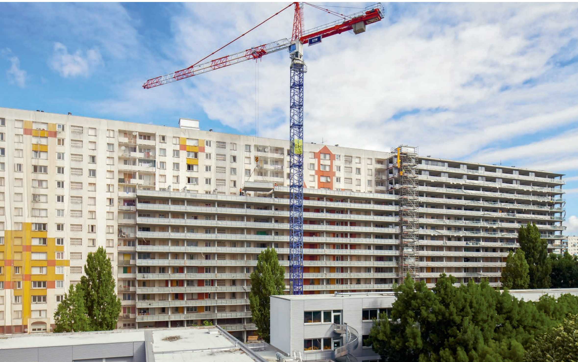
Grand Parc, a postwar social housing complex consisting of three buildings, was to be demolished. The architects proposed to keep the existing structure and extend it instead. The cost of the transformation was roughly half as much as the erection of new apartment buildings.
