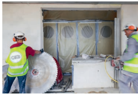
The tenants were able to stay in their dwellings during the short periods of construction works that were achieved in only 12–16 days per unit, thanks to prefabricated modules. Furthermore, rents were not increased after the transformation.
