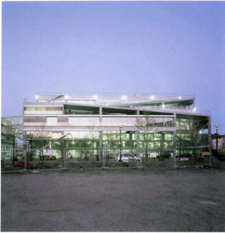
The three decks – at nine, sixteen and twenty-two metres above ground level – are connected by a sloping external ramp leading to the roof.
