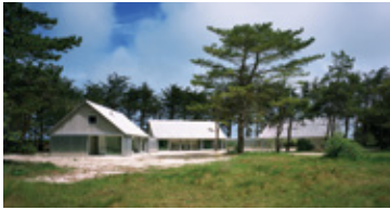
House at Keremma, Tréfléz Completion 2005 Client Private Program Individual house Area 316 sqm Cost 260 000 € net
