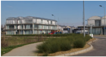
Social housing, Trignac, Saint-Nazaire Completion 2010 Client SILENE Saint-Nazaire Program 23 renting social dwellings Area 2 852 sqm SHON Cost 2,3 M € net
