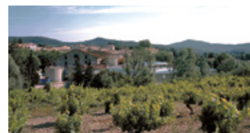
Cellar and wine storehouses, Embres et Castelmaure Completion 2007 Client Cooperative cellar of Castelmaure Area 2 000 sqm new and 400 sqm existing renewed Cost 1,1 M € net
