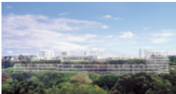
Éco-Quartier, La Vecquerie, Saint-Nazaire Competition 2009, non prize winner Client Silene, OPAC Saint-Nazaire Program 153 dwellings and greenspaces Area 16 700 sqm housing (including wintergarden) Cost 15,3 M € net (including VRD, car parking and greenspaces)
