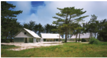
House at Keremma, Tréfléz Completion 2005 Client Private Program Individual house Area 316 sqm Cost 260 000 € net
