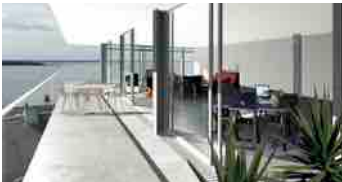
Social housing, St Nazaire Competition 2004, non prize winner Client Silène - OPAC Program 55 dwellings (27 existing transformed, 28 new) Area 5,117 sqm usable space, 66 apartments (from 66 to 141 sqm) Cost 3,39 M€ net
