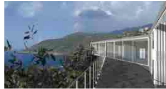
House in Morsiglia, Corsica Project 2001, unbuilt Client Private Program Individual house Area 370 sqm (240 sqm living space + 130 sqm terrace) Cost 200 000 € net
