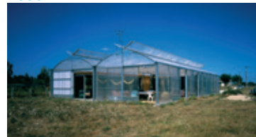
House in Coutras Completion 2000 Client Private Program Individual house Area 290 sqm Cost 64 800 € net (2000)
