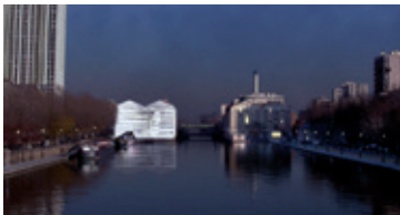
Commercial and leisure time building, Paris la Villette Competition 2004, non prize winner Client ING Real Estate, France Program Shopping mall, activities, offices, leisure, 24/24 Area 13 500 sqm Cost 11,5 M€ net
