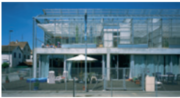
Social housing, Mulhouse Completion 2005 Client SOMCO Program 14 apartments in a project of 61 apartments built by 5 architect's teams Area 2 262 sqm Cost 1,05 M€ net (75 000€ net each house)
